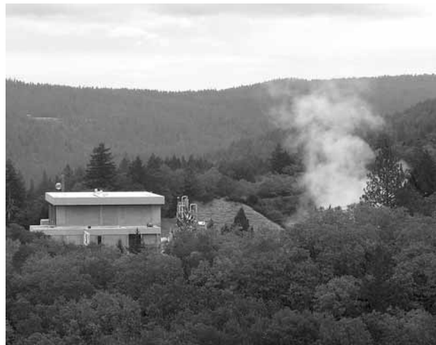
Bottle Rock Power Plant
